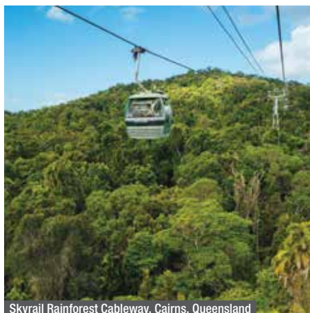
Skyrail Rainforest Cableway, Cairns, Queensland
